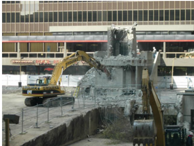
Stage demolition and work in the east grove
