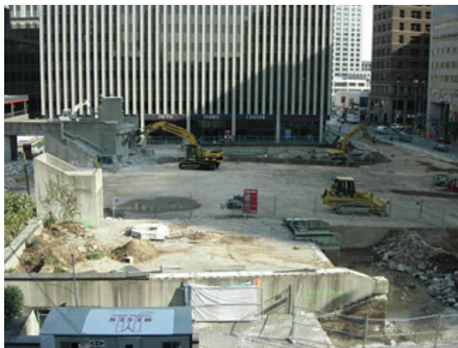
View of progress on the Square from Vine Street facing east
