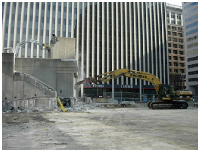
Demolition of the stage and associated elevator shaft
