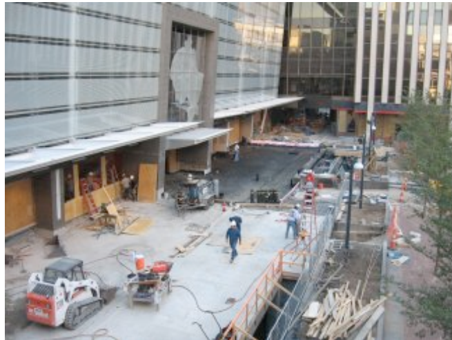
Work in progress - view from Via Vite Restaurant
