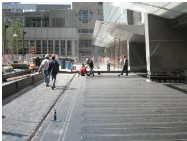
Work in progress - view from the Fifth Third building
