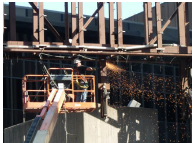
Work begins to remove steel support structure from the stage.
