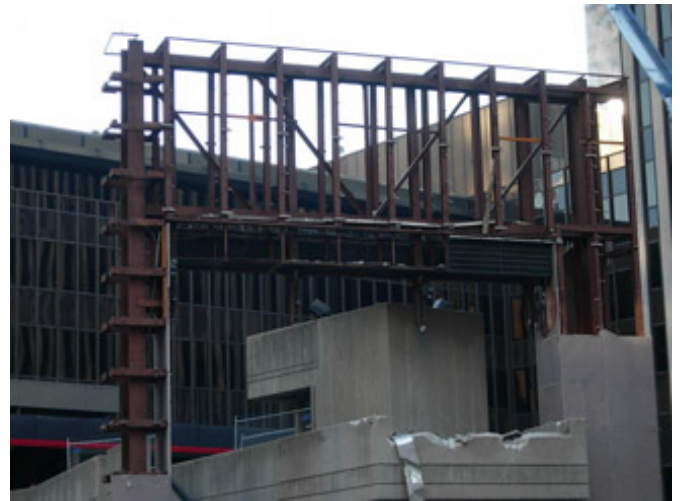
Granite slabs removed.
