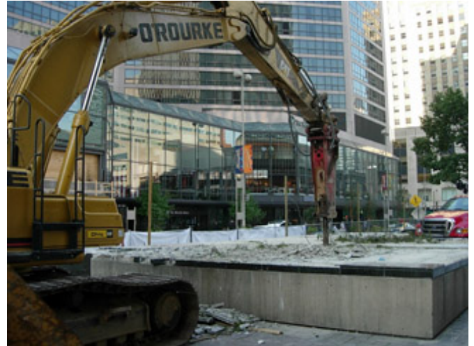
Excavation on the base of the Westin Skywalk stairs.
