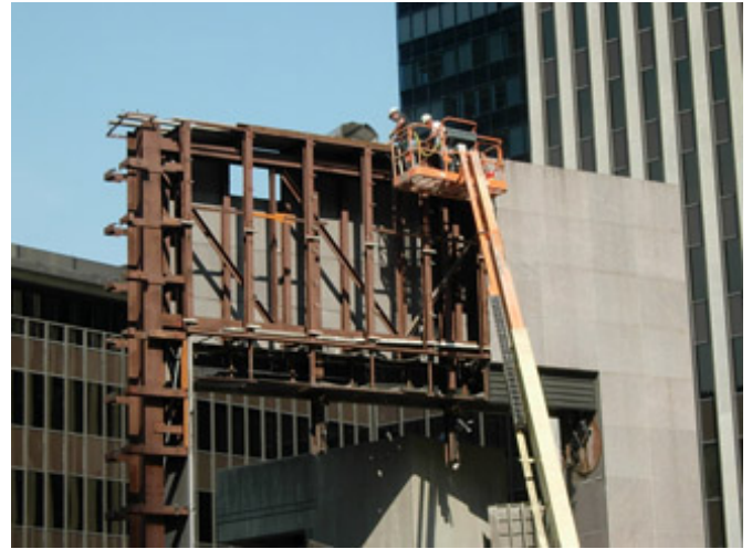
Workers remove granite slabs from the stage.
