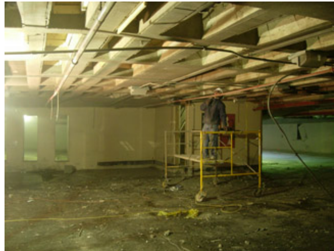
Workers prepare the garage for structural concrete repairs
