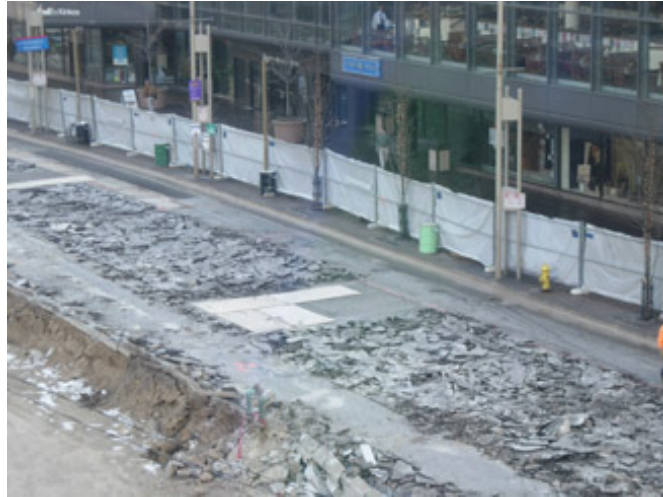
Closer view of demolition on 5th Street
