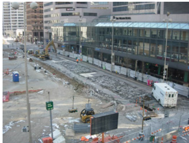
Overhead view of demolition work on 5th Street
