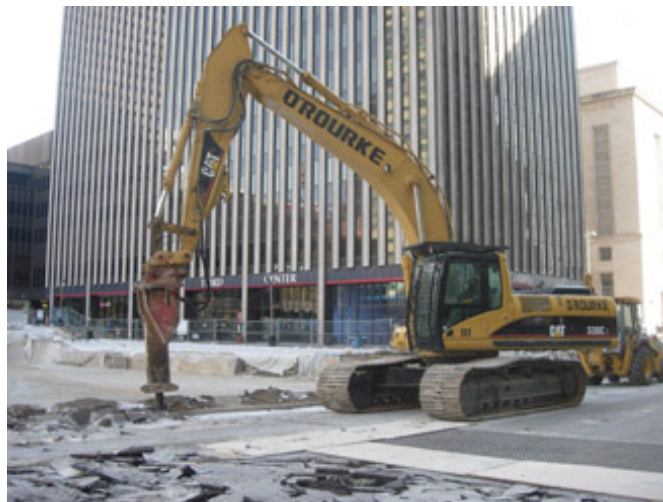
Demolition of the curb along 5th Street
