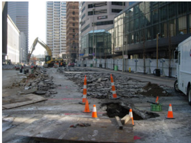
Street level view of work on 5th Street
